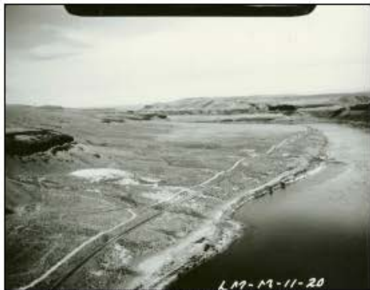
Photo 1. Right Bank, 55 Mile area, 1968 oblique.
