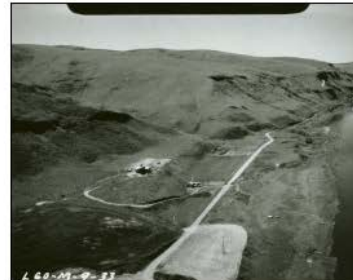
Photo 3. Right Bank, Penawawa area, 1958 oblique.
