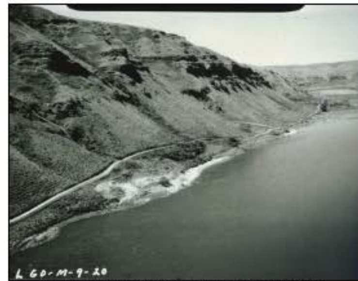
Photo 2. Left Bank, Shultz Bar area, 1968 oblique.
