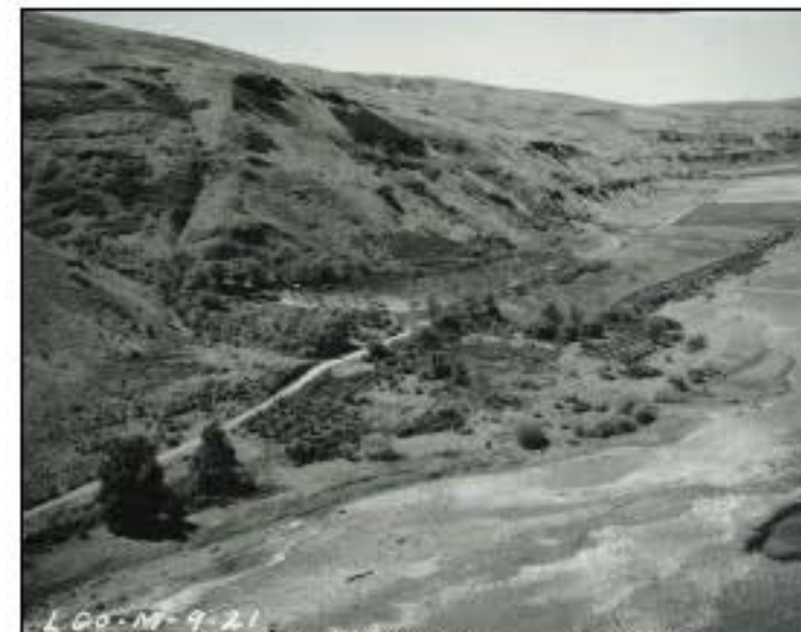
Photo 3. Left Bank, Shultz Bar area, 1968 oblique.
