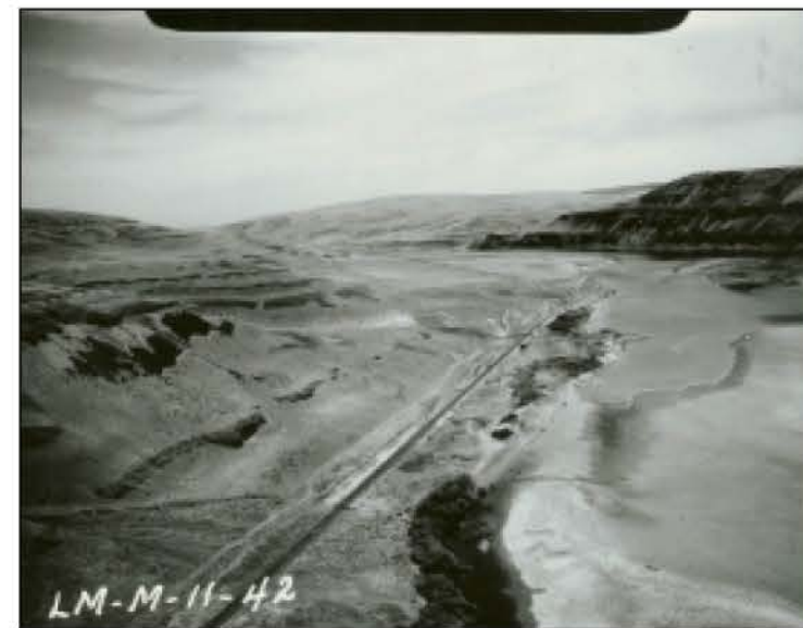
Photo 2. Right Bank, Goose Island area, 1958 oblique.
